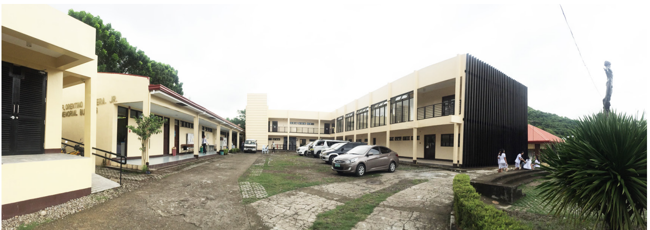
SHS Palo Leyte Administrative Building, completed in September 2016
